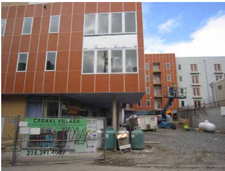
Cedars Village, 60 units of senior housing, during construction
