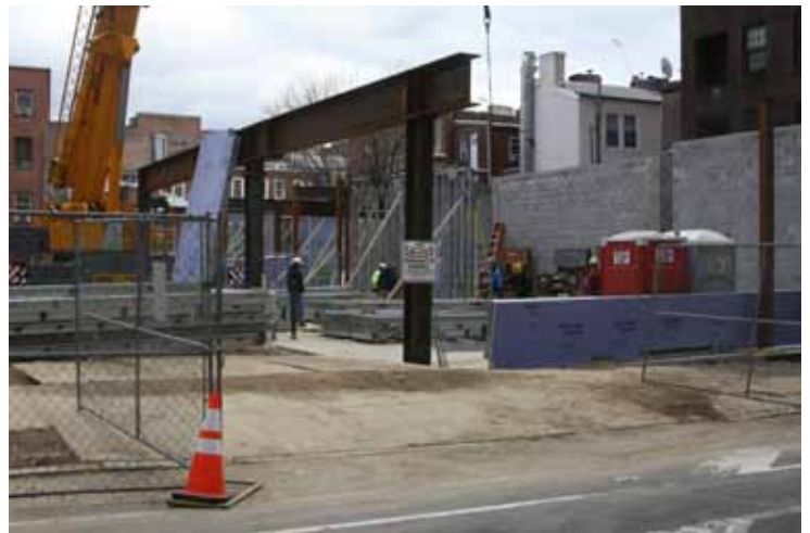
John C. Anderson Apartments, 56 units of senior housing, under construction
