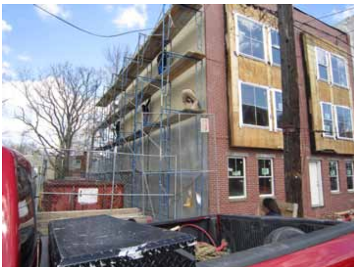
3909 Haverford Avenue during construction
