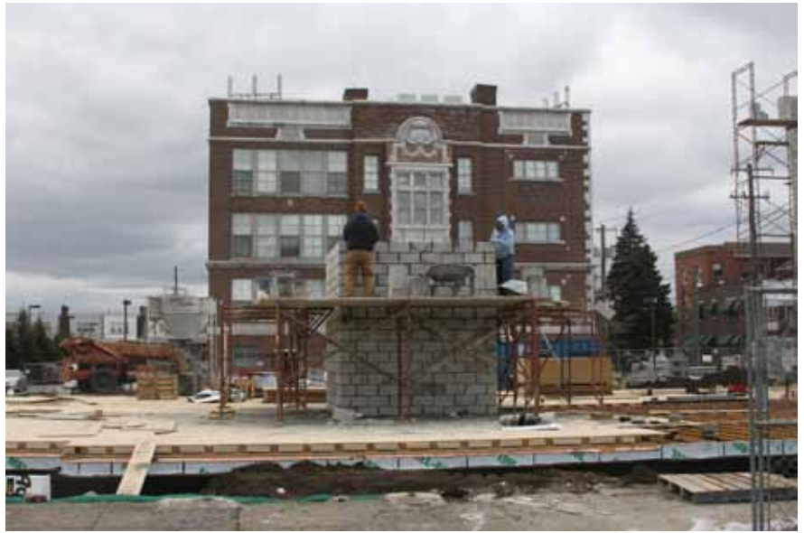
Anthony Wayne II, 46 units of rental senior housing, under construction
