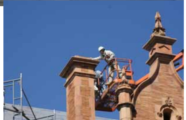
Nugent Senior Apartments renovation
