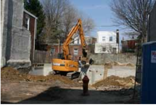
Beaumont Accessible Homes under construction
