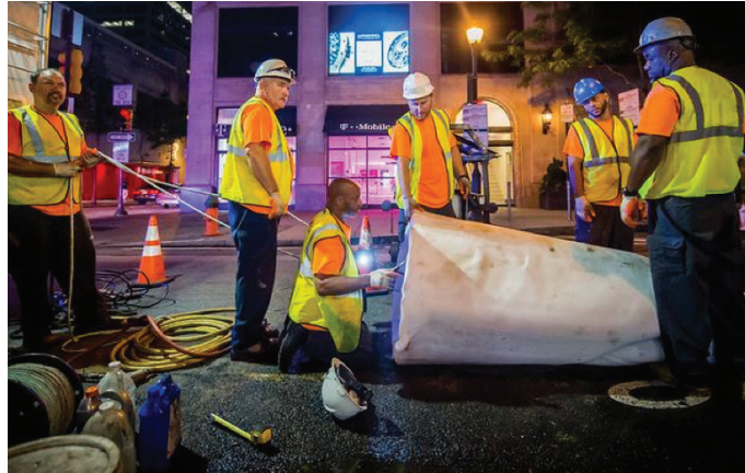
PWD EMPLOYEES WORKING ON A SEWER RELINING PROJECT
