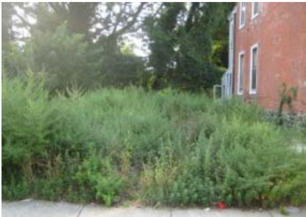
Vacant property before cleaning (8/21/2010)
