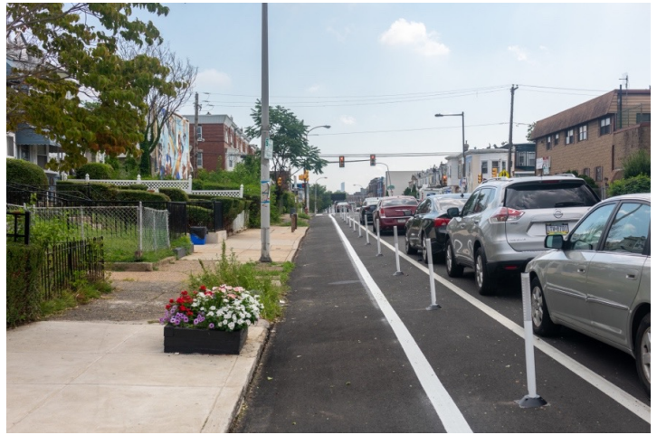
A VIEW DOWN THE NEWLY INSTALLED PARKING SEPARATED BIKE LANE ON CHESTNUT STREET NEAR 61ST STREET. WITH THIS LATEST ADDITION, CHESTNUT'S PARKING SEPARATED BIKE LANE NOW EXTENDS NEARLY 4 MILES FROM 62ND STREET TO 22ND STREET.
