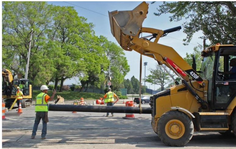
PWD crews replace a water main to ensure that the city's 3,000-mile network of water mains provides reliable delivery of safe, top-quality drinking water.
